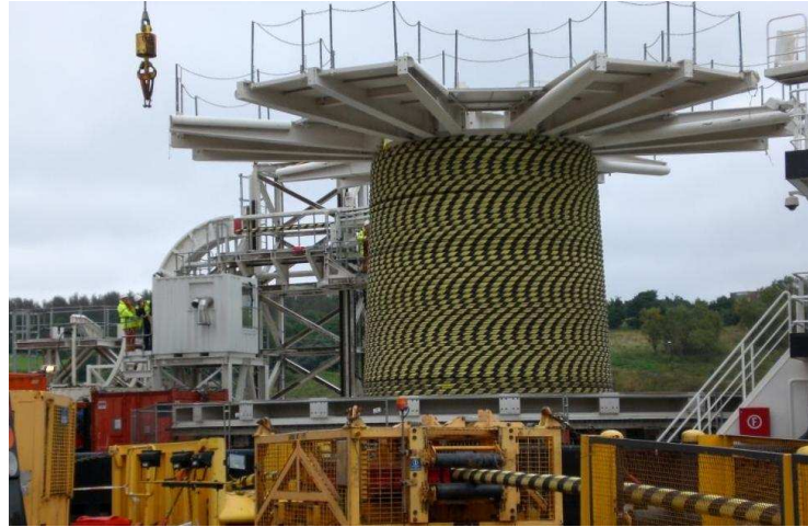
20Te Capacity Lay System with 2200Te Reel
