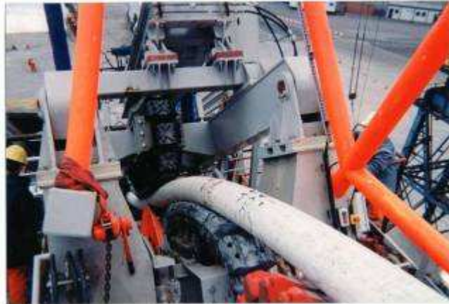
16"NB Pipe Straightener – Subsea 7 Skandi Navica
