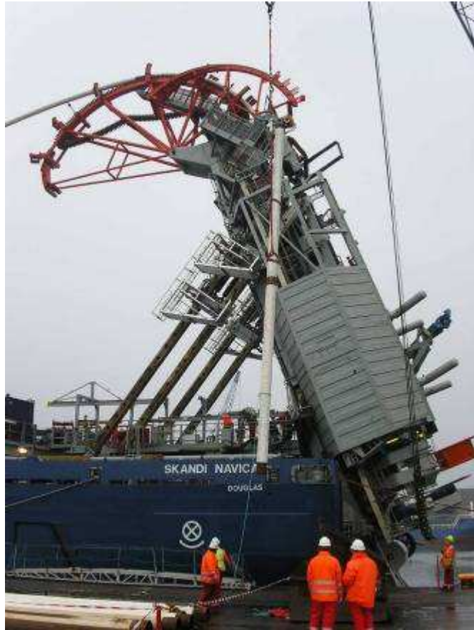
Pipe Straightening trials on the Skandi Navica
