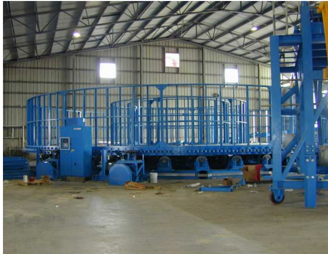
1000Te Umbilical Carousel Installation - Texas USA
