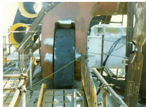
Jacket Clevis with Lifting Beam installed and Lift Pins engaged.
