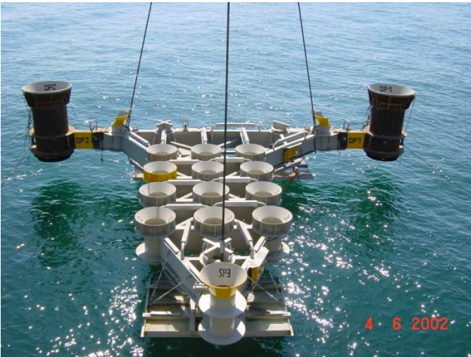
Typical Drilling Template being lowered to the seabed.
